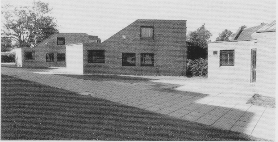
5.35 University of Warwick: Whitefields student residences, by Goodman and Short 1972–3. Each house contains twelve single study bedrooms and a communal kitchen and bathroom.
