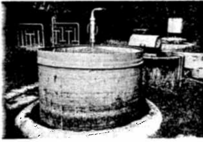
Fig. 3.4 A Typical Bio-Gas Plant Installation.
