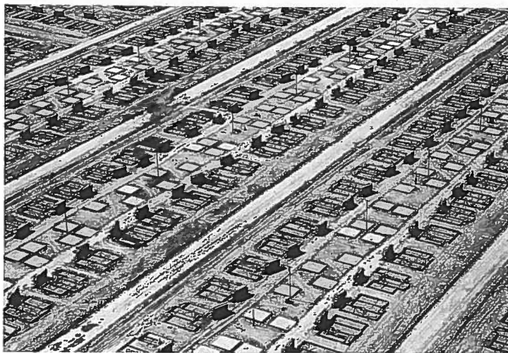
29 William Garnett, four views of a California tract under construction: after bulldozing; after house and garage foundations were poured; during framing; and as salable space. (Copyright, William Garnett, 1955)
