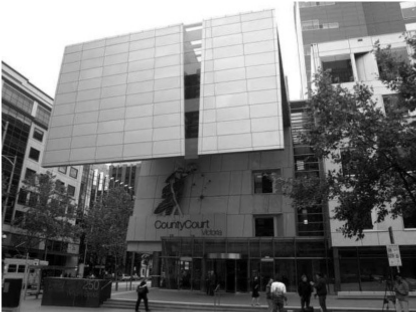
Figure 8.4 County Court, entry.
