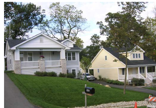
4. Habitat Houses. Judson University "Community Service" class "live" project, Elgin, IL, modelled after Sears Kit Homes from circa 1920. Design Critics: David Amundson and Nathaniel Brooks, 2003. (Photo by Marga Jann.)
