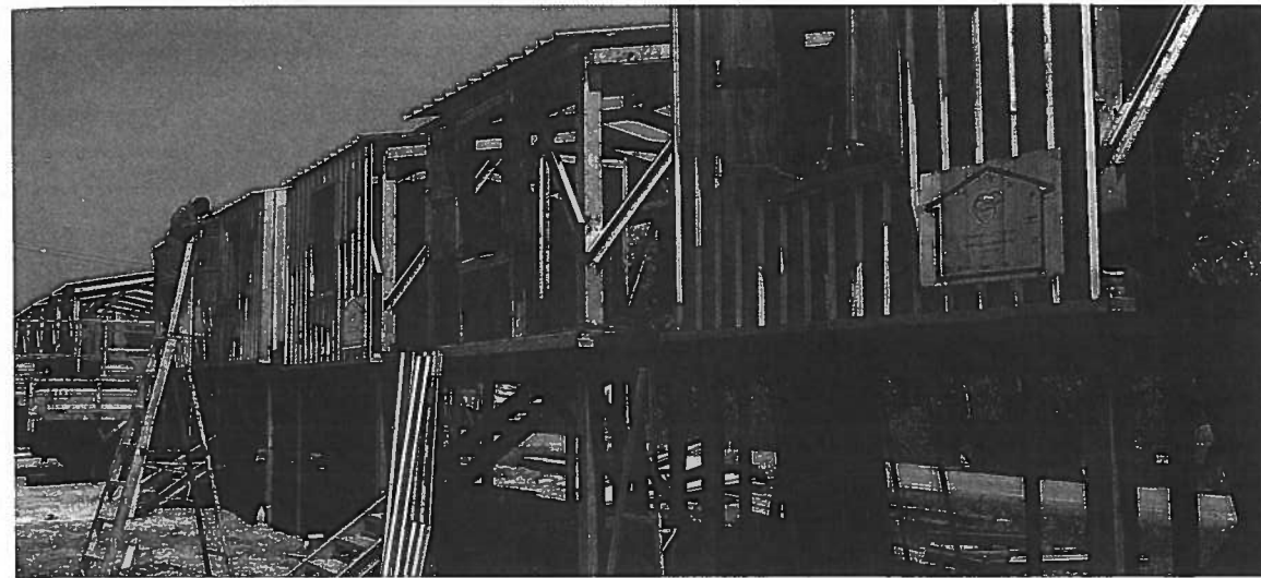
The Engineering Unit of the Thai Army erected temporary housing in Ban Nam Kaem, Takua Pa province, Thailand, following the Indian Ocean tsunami of December 2004.
